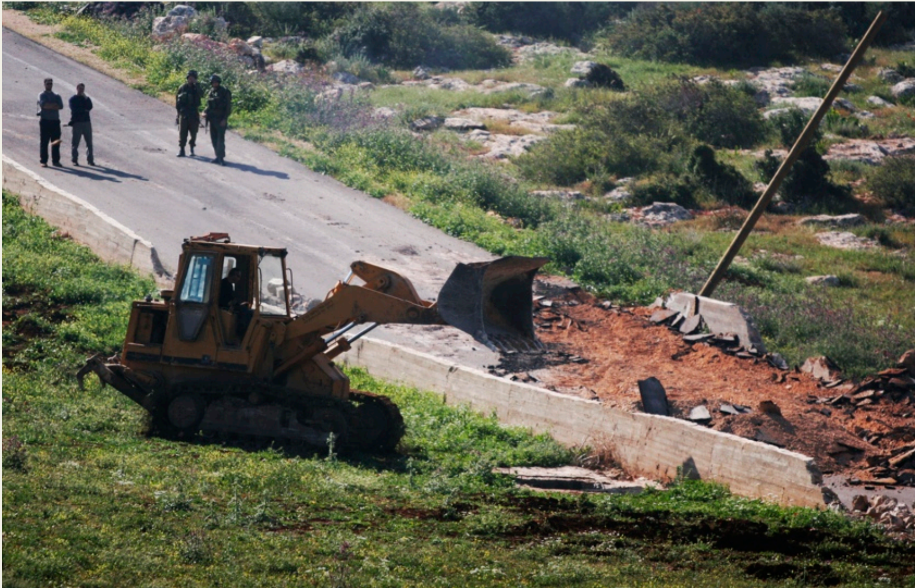
April 7, 2011: Israeli Army Demolition Bulldozers destroy Peace Road and two small homes with animal stables
