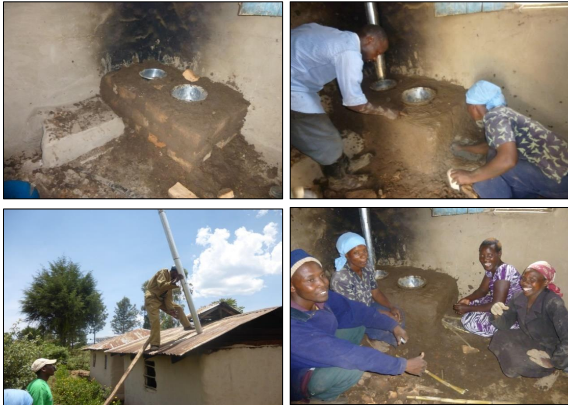
Various stages involved in installing a smokeless stove
