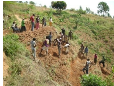
7/09 Terrace building begins
