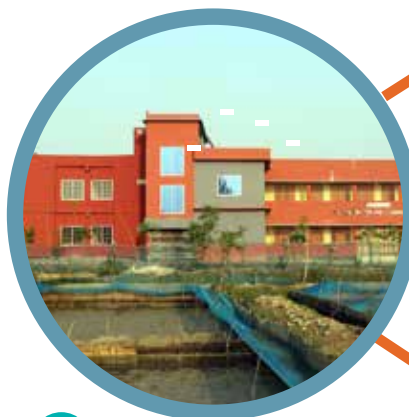
2 Established Cyclone and Training Shelter
